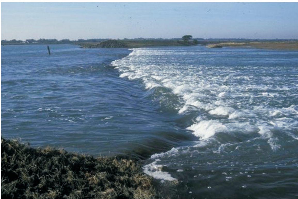
Breaching of sea wall 2002
