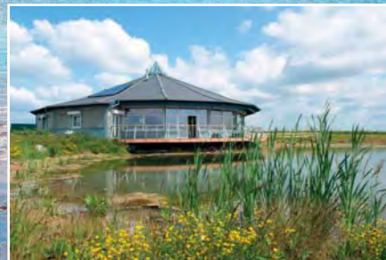
Abberton Reservoir Visitor Centre
