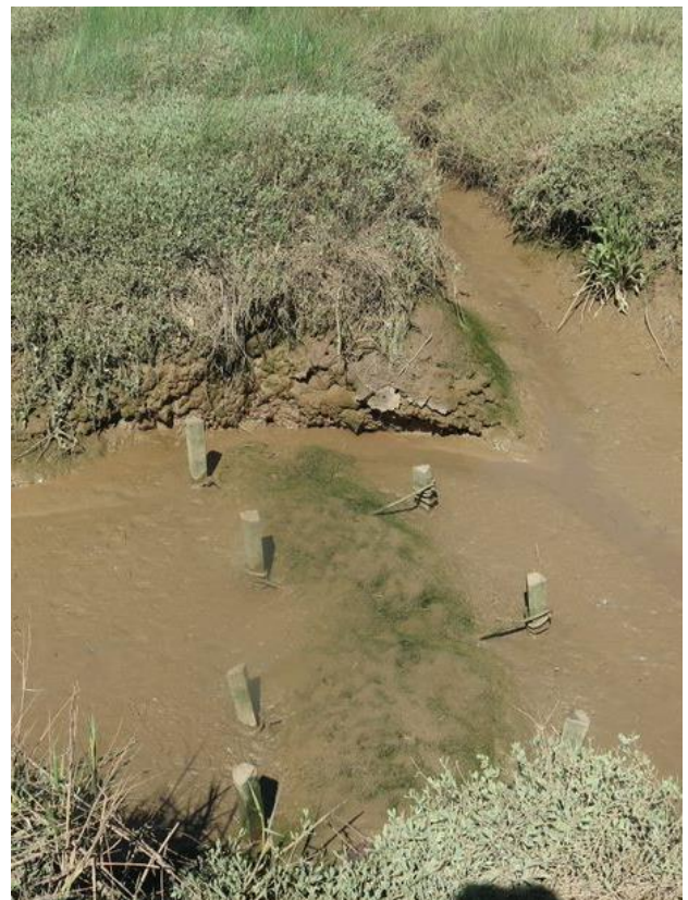
Figure 9 Moverons structure 5 in June 2020 (left) and June 2021 showing how the structure has 'bedded in' to the channel.
