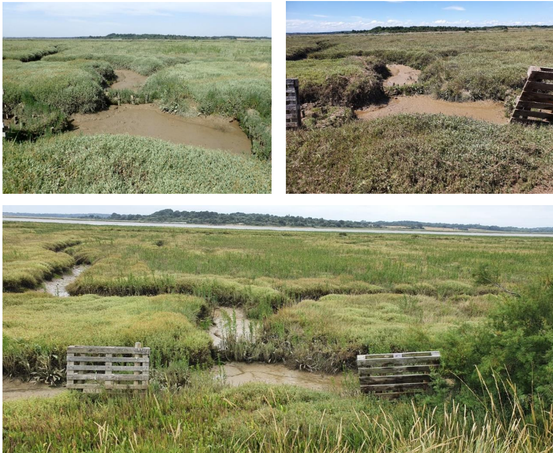
Figure 11 Moverons structures 6, 7 and 8 in (A) August 2019; (B) June 2020; (C) June 2021 showing how vegetation has established on the structures . NB the palettes have been erected to prevent sheep traversing onto the marsh via the structures.
