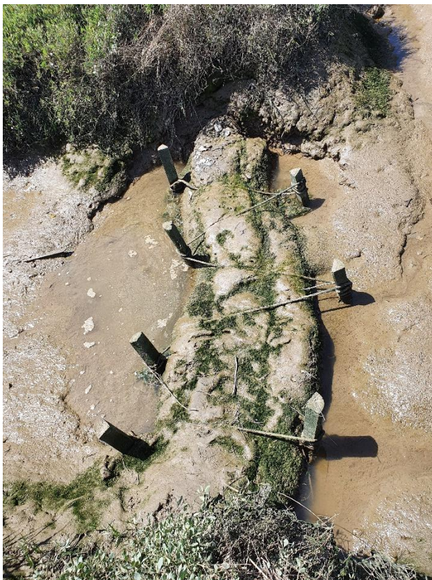
Figure 9 Moverons structure 5 in June 2020 (left) and June 2021 showing how the structure has 'bedded in' to the channel.
